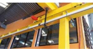
To choose the most suitable line required for a certain current and to define the location of the supply point/s, add up all the currents of any motors that could be in simultaneous operation, as well as any foreseeable voltage drop.
