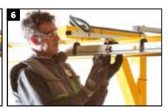
Cover the connection, sliding the **joints RGMM02** (**both halves**) (Photo 6) until completely closed (**click**) using the pressure tabs (Photo 7).
